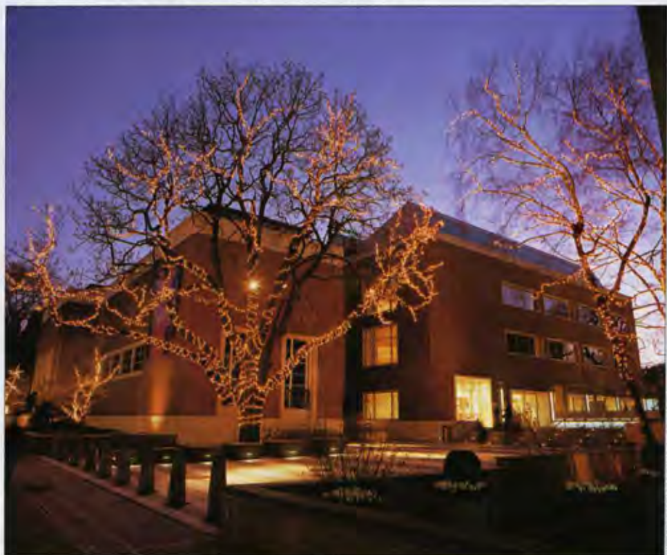
The Portland Art Museum's recently completed renovation and construction, by Ann Beha Associates, includes the new 60,000-square-foot Hoffman wing.
