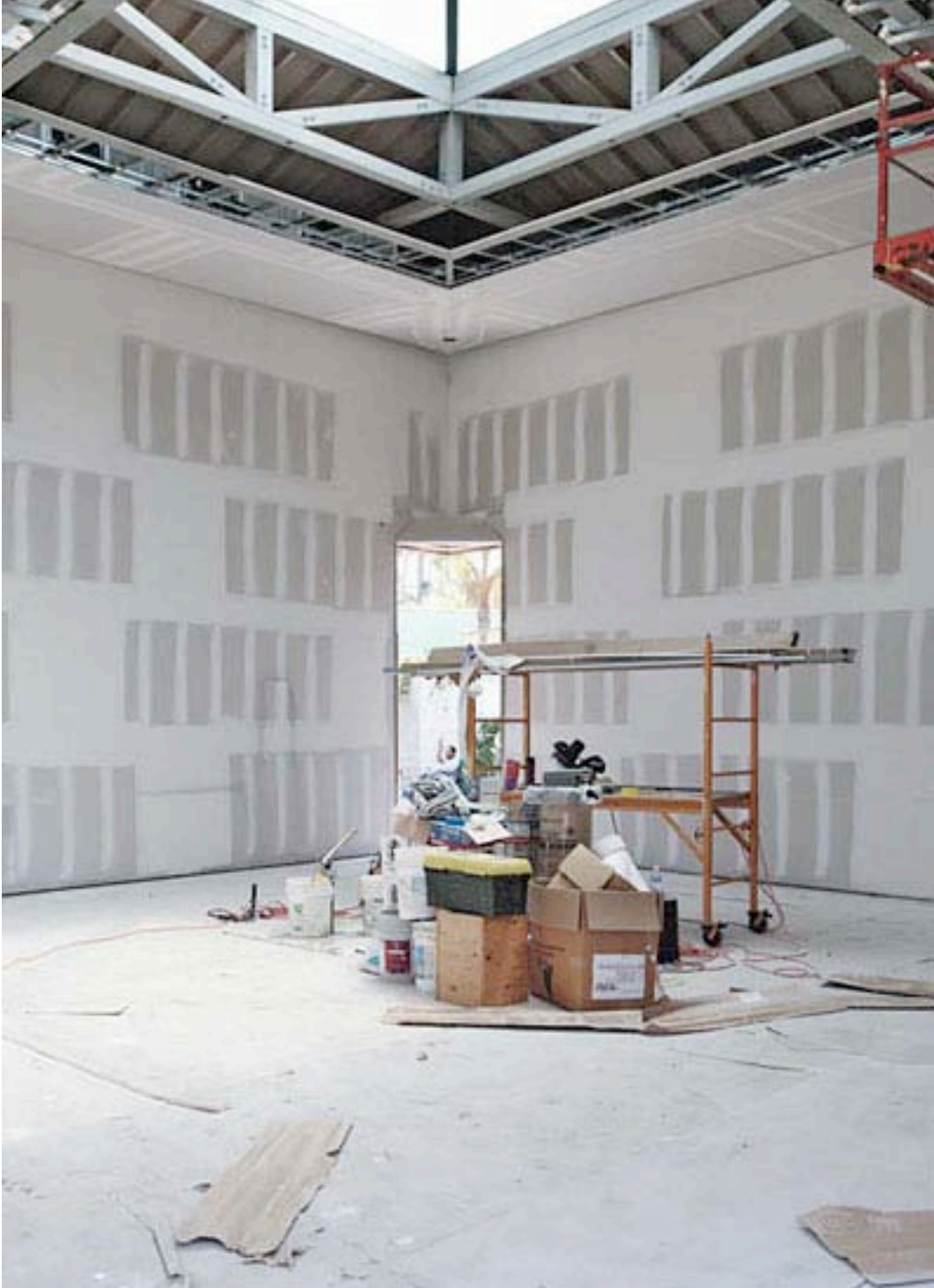
Construction at L&M Arts Photographed by Jason Schmidt August 2010
