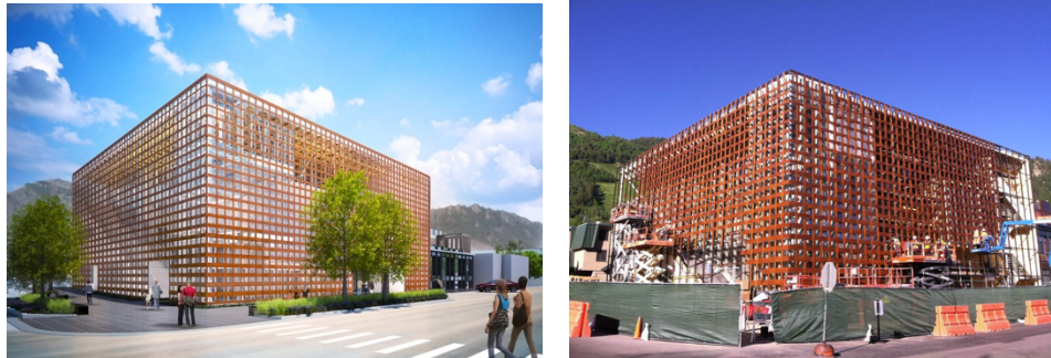
Left: Rendering of New Aspen Art Museum. Image courtesy of Shigeru Ban Architects. Right: Photograph of New Aspen Art Museum under construction. Image courtesy of Aspen Art Museum.
