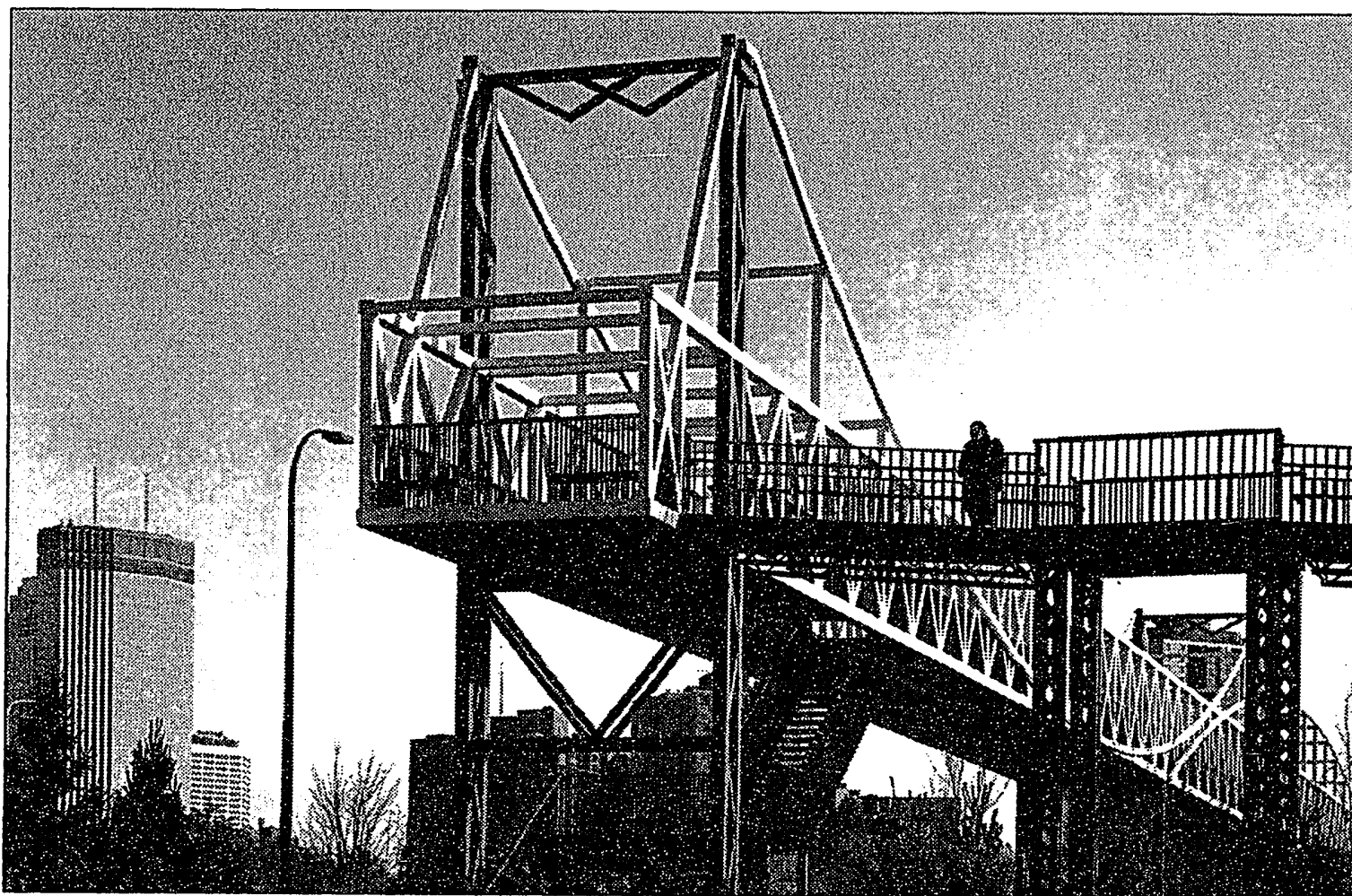
The bridge to the Minneapolis Sculpture Garden—a loving tribute to the two great types of bridge, suspension and truss
